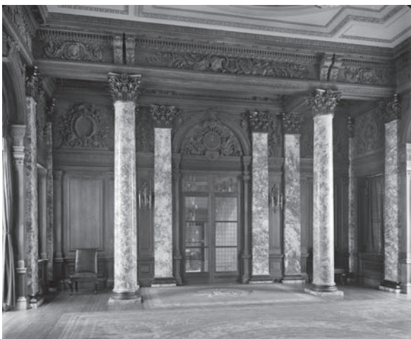
Above The library, east end, July 1918.
